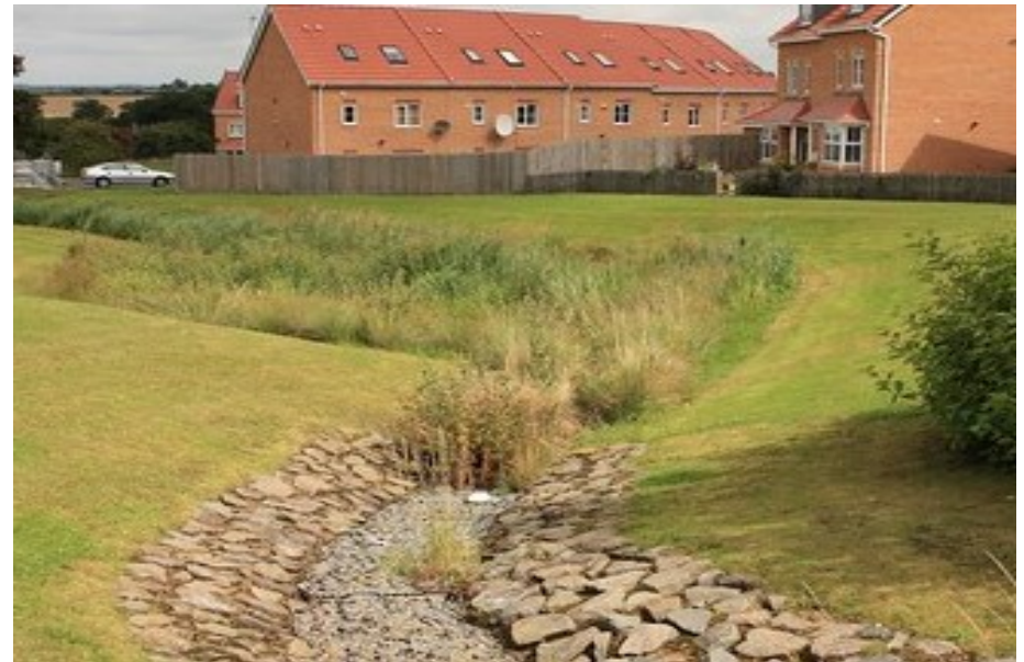
SuDs scheme for a residential development – Susdrain.org
